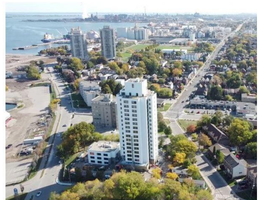
Ken Sobel tower is the tallest retrofitted Passivhaus in the world. Photo by Codrin Talaba
